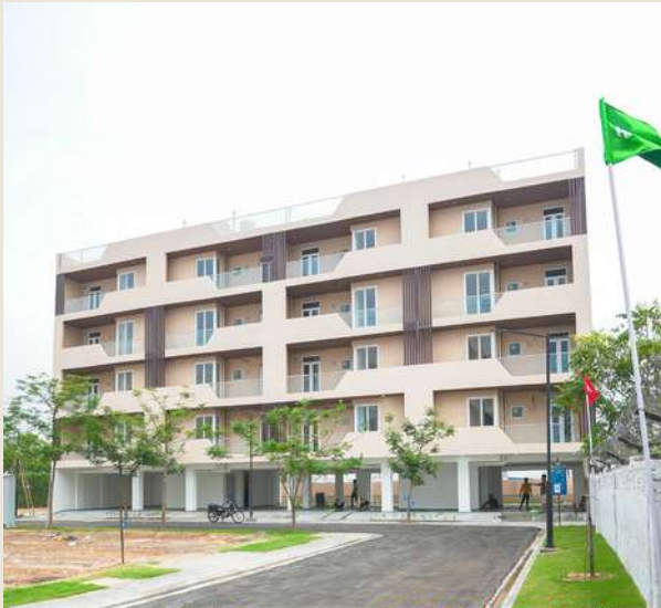
SHF Floors- Facade
